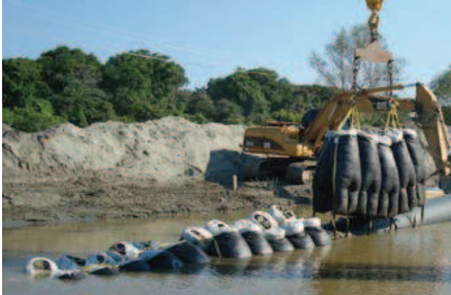
Wet installation of a 42" 14,000 lb PipeSak
