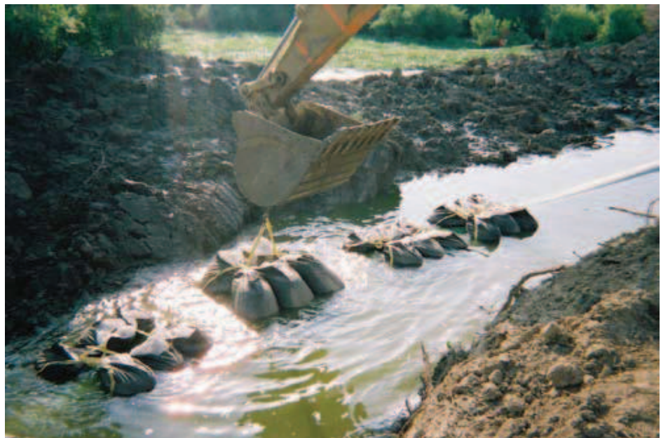
Sinking 36" pipe with multiple 9,000 lb PipeSak
