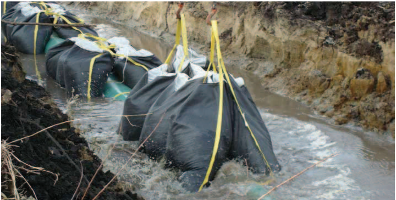
Wet installation of a 36" 9,000 lb PipeSak
